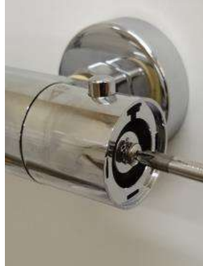
2. Using a X-head screwdriver remove the Temperature Handle.
