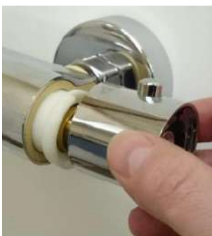
7. Once the Shower is set to the desired temperature, relocate the Temperature Handle onto the Cartridge spline, ensuring that the Over-ride Button Pin is against the Temperature Stop Lug. (This prevents the temperature from exceeding 38°C unless the Over-ride button is pressed)
