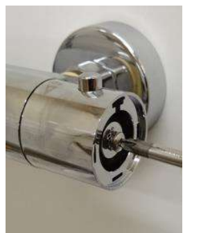
8. Again using a X-head screwdriver secure the Temperature Handle.
